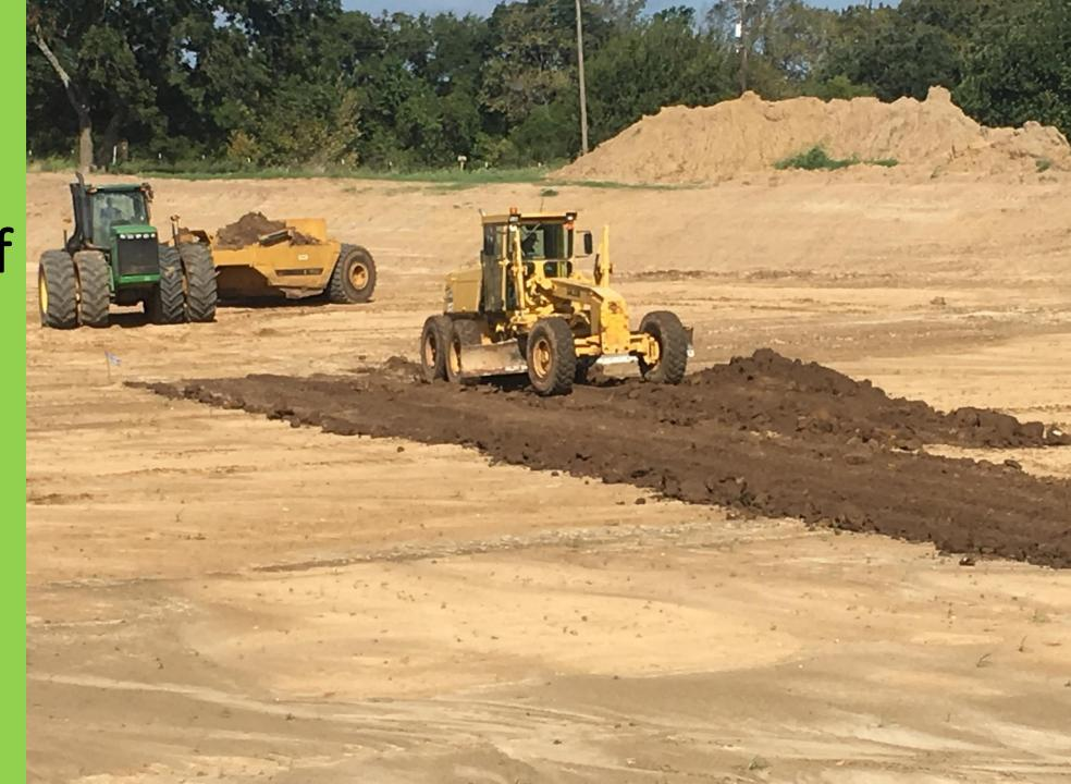
Rome Plowing ... cuts to 14 inches in depth. Mixes topsoil and levels the ground.
