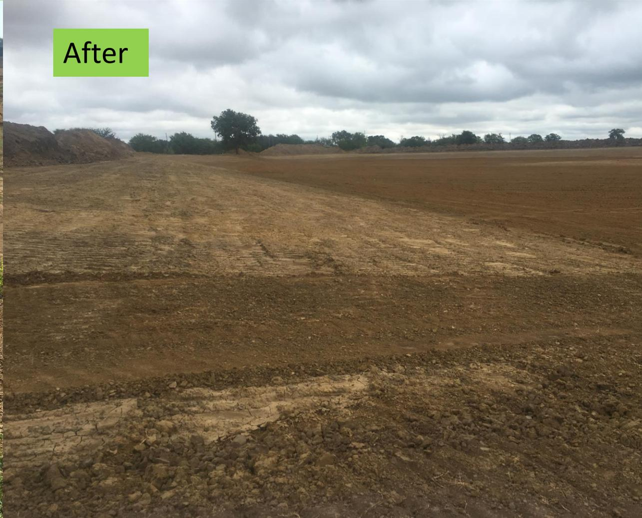
**Final Leveling on the top of the slope. Berm is placed at the top to prevent water from entering into the pit (that would cause erosion).**
