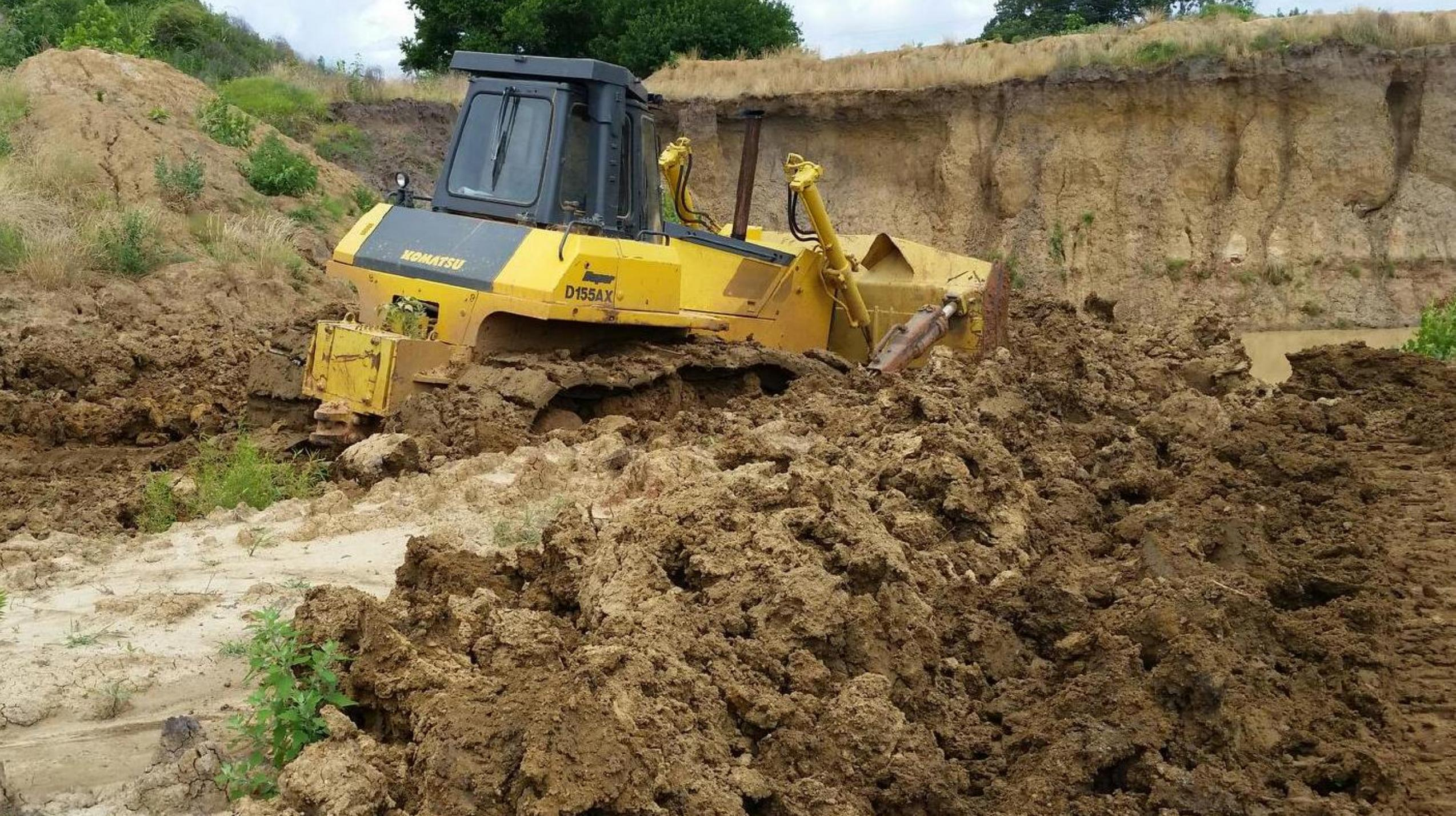
To Safely get our slopes workable, experienced operators on Excavators and Dozers leveled the slope.
